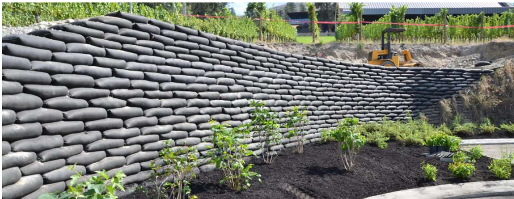
Figure 4.18: Vegetated green wall retaining solution, prior to vegetation growth
