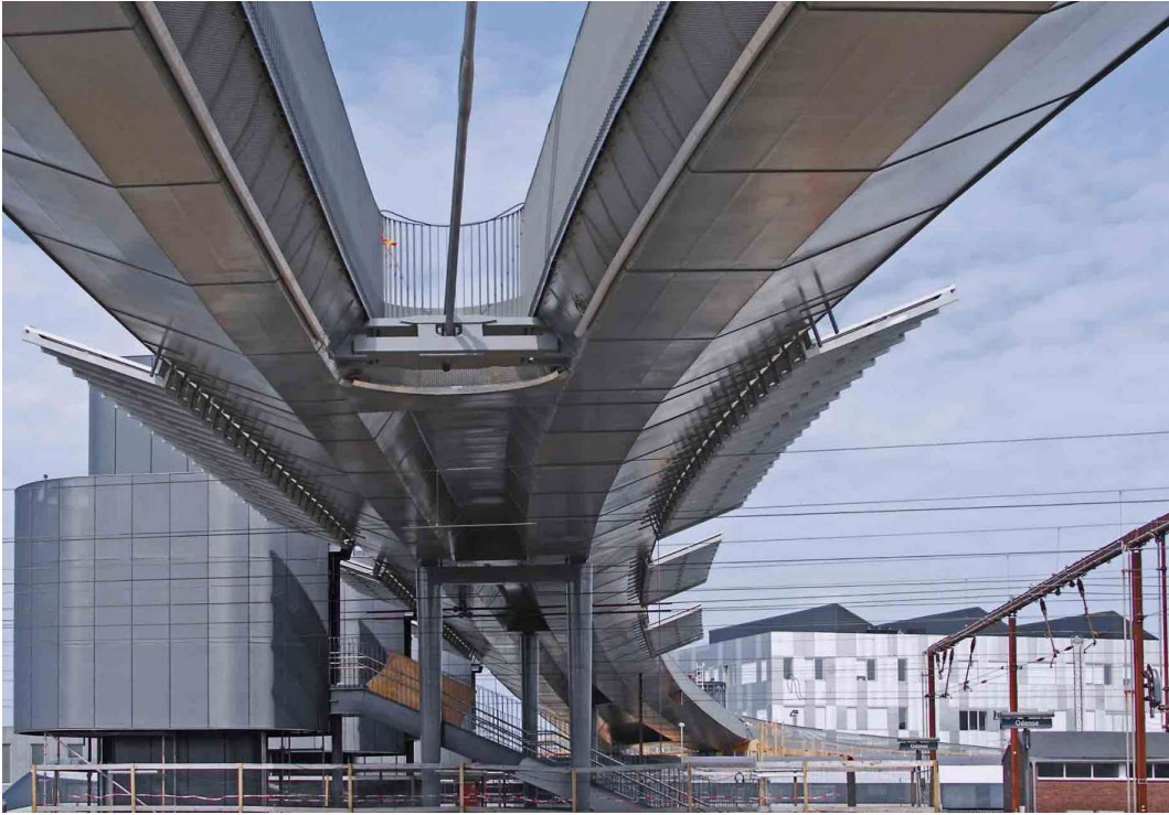
Figure 11 Example of under bridge screening on new pedestrian and cycle bridge in Odense, Denmark with 1.2m high parapets with vertical bar infill
