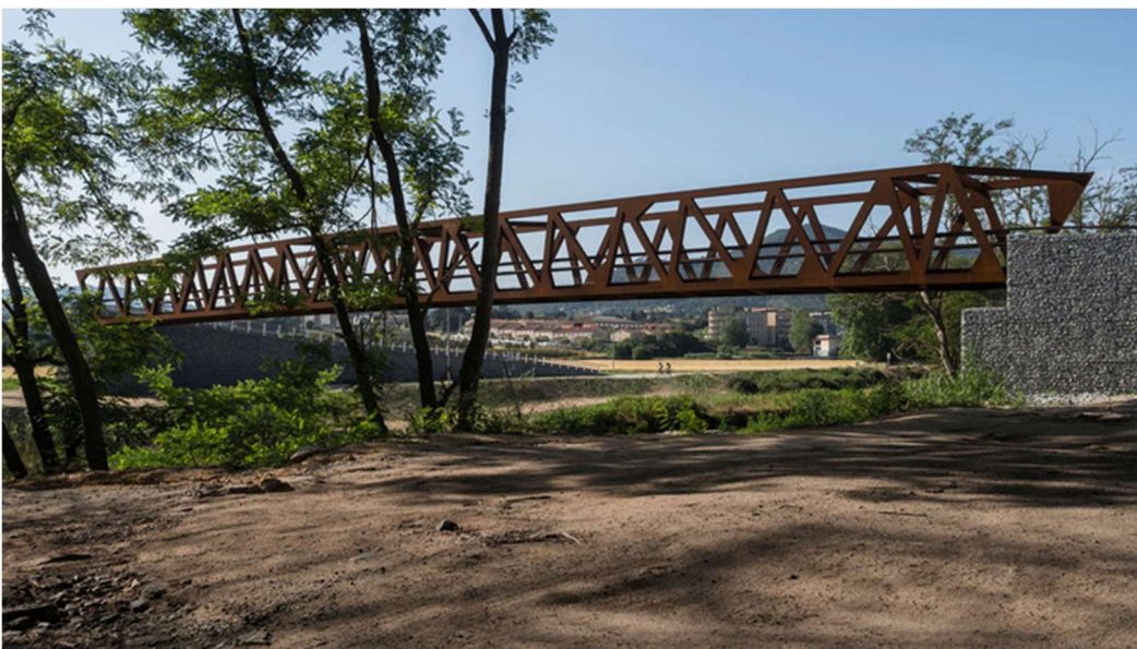
Figure 4.4: Example of through truss pedestrian and cycle bridge of higher aesthetic (note weathering steel not expected applicable for this project, architectural option would be painted steel)
