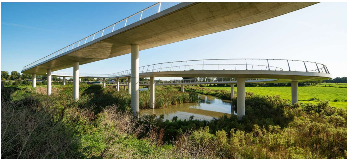
Figure 4.15: Example of reinforced concrete elevated ramp structure with monopiles/columns (northern approach ramp)
