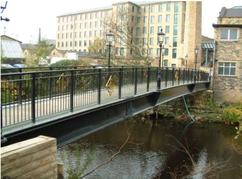
Figure 4.13: Steel edge beam bridge
